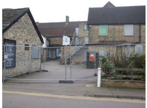
Church Street – fencing across car park entrance
